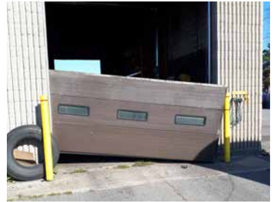
Wash bay door blown off
