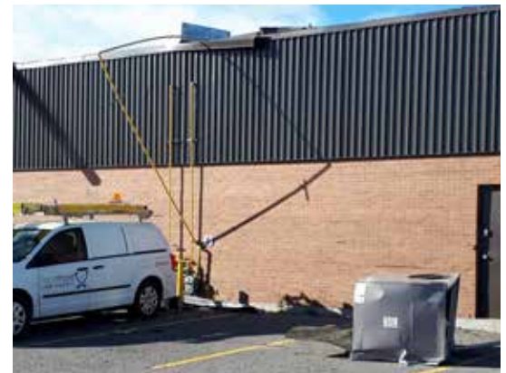
A/C unit that blew off neighbour's roof
